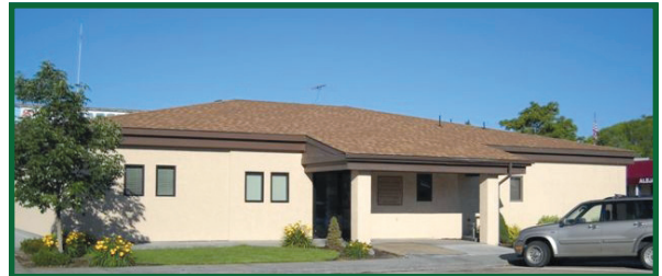
New façade of Terry Reilly's clinic expansion in Marsing blends in with rest of building.
